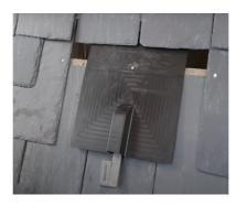
Put solar flas h on the bracket, cut the trims according to the tile size
