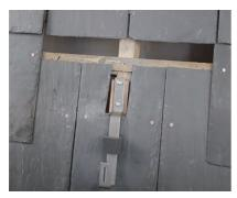
Remove the tiles on remarked position, shims to increase height if necessary, then fix the hook and foam to the bracket drop
