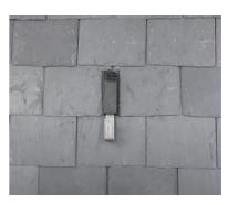
Cut tiles and recover to the solarflash
