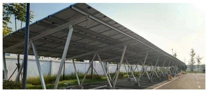
Solar carports are structures that provide shade to parked cars while also harnessing solar energy through the use of solar panels installed on the roof. They are typically constructed using sturdy material such as aluminum and are designed to withstand the weight of solar panels and other environmental factors.
